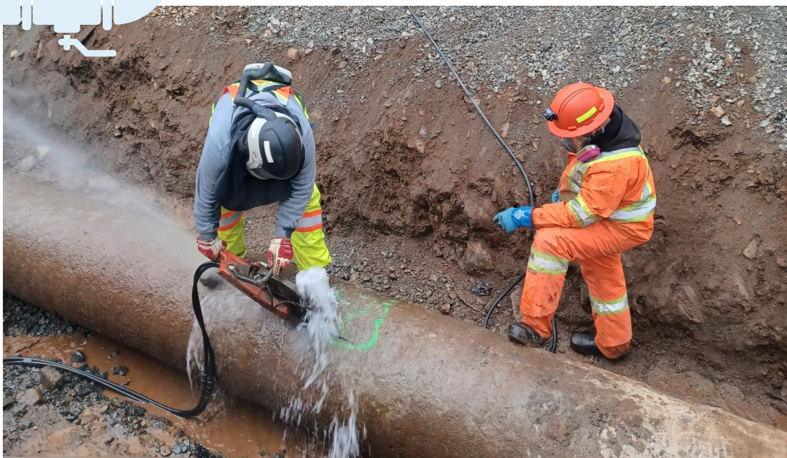
Halifax Water crews repair water mains to reduce water loss, restore service, and improve reliability for customers.
