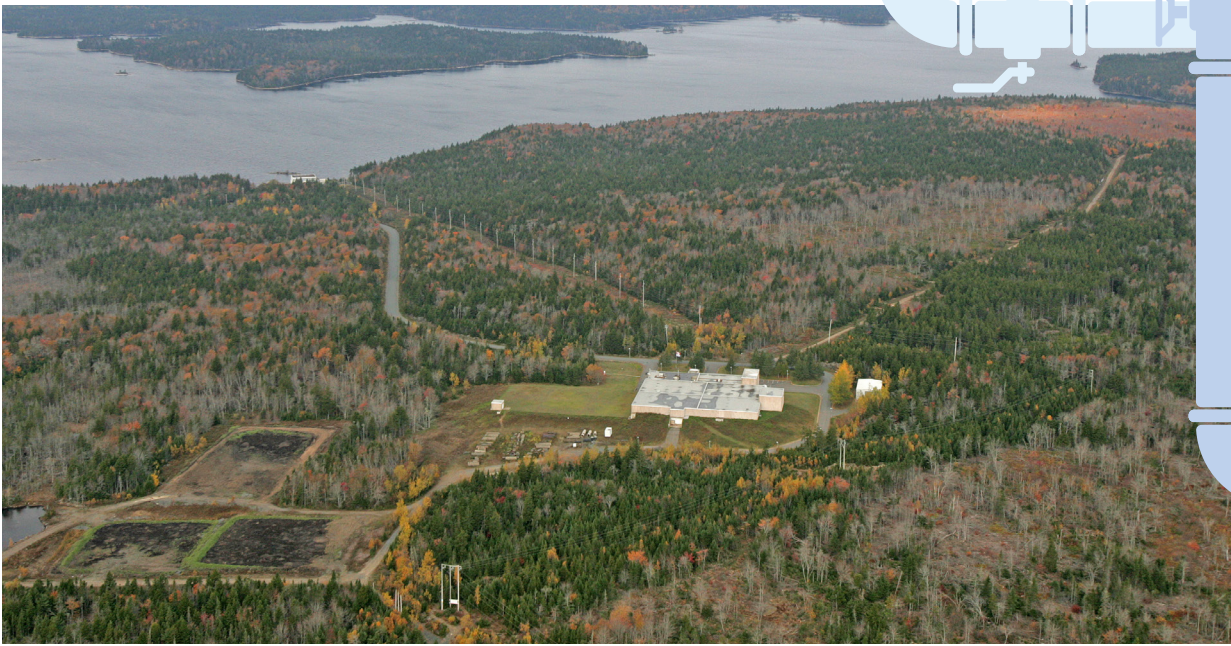
The J.D. Kline Water Supply Plant is a focus of operational resiliency work to strengthen reliability, redundancy, and emergency preparedness.
