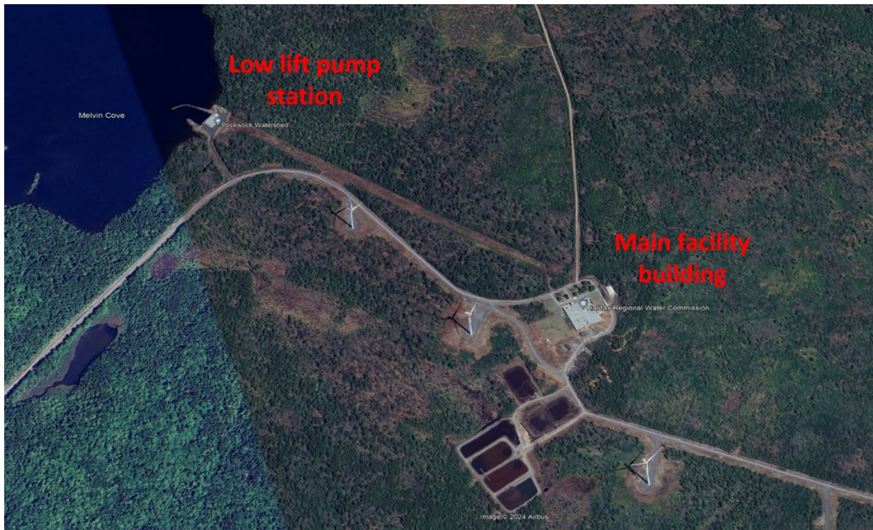
Figure 2-2: Aerial Photograph of the JDKWSP indicating the low lift pump station and the main treatment facility building.
