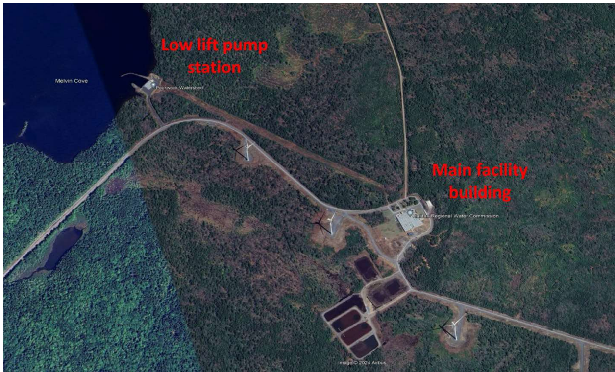
Figure 2-2: Aerial Photograph of the JDKWSP indicating the low lift pump station and the main treatment facility building.
