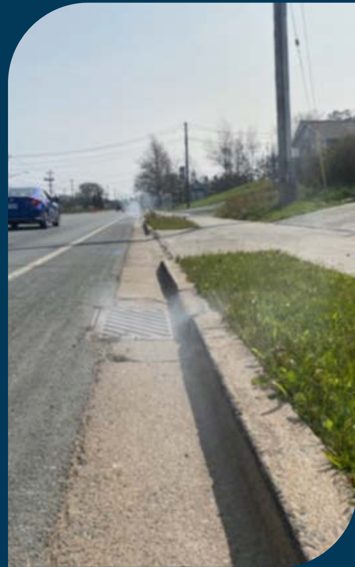
Catch Basin smoke test
