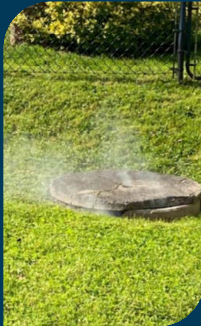
Manhole smoke test
