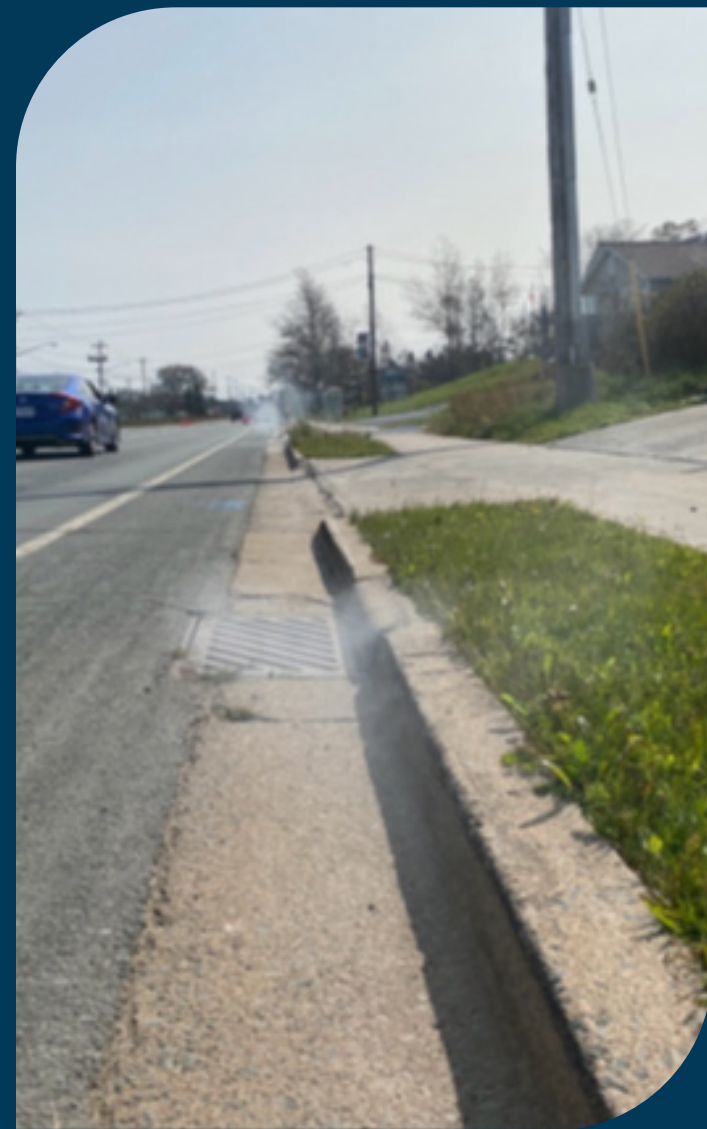
Catch Basin smoke test
