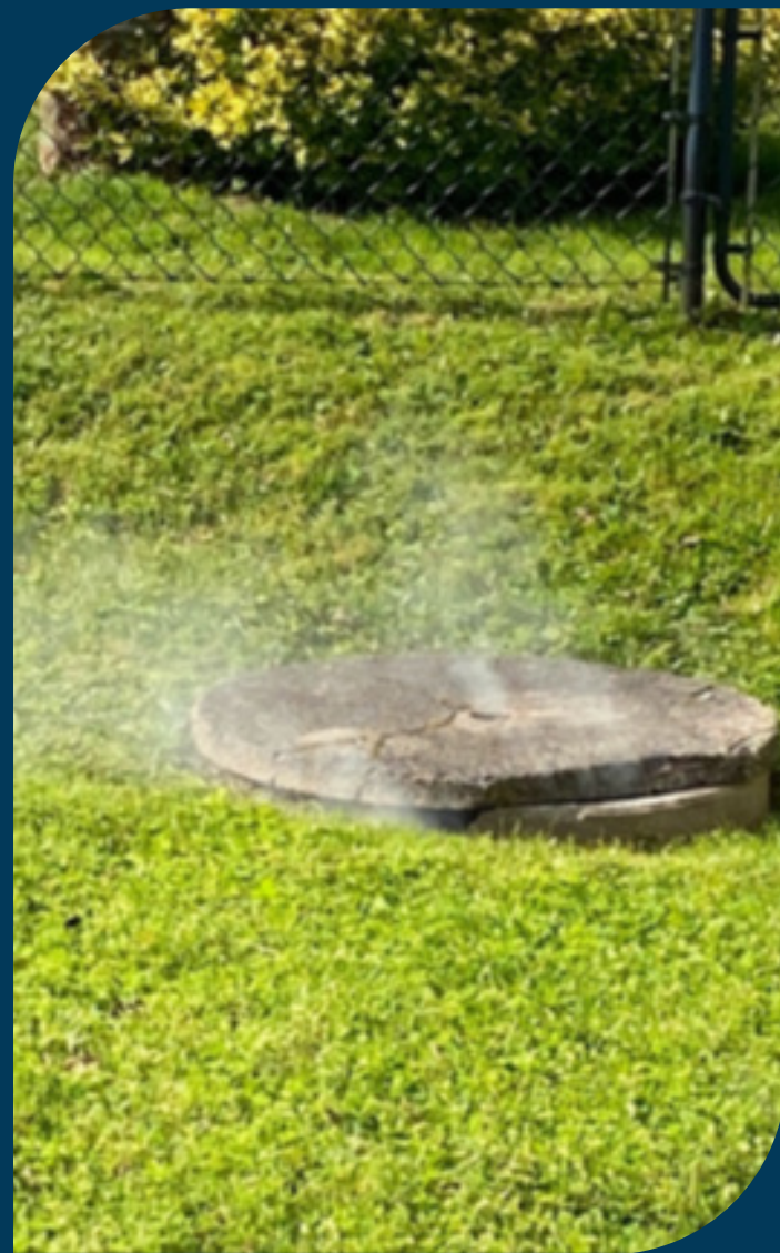
Manhole smoke test
