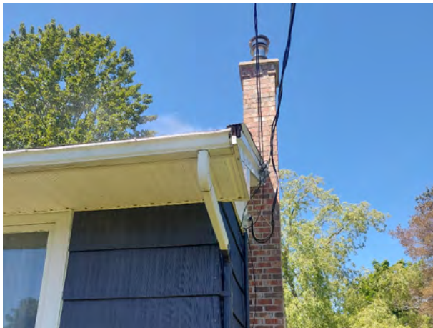
Private downspout smoke test
