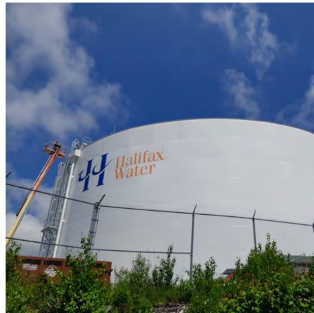
Akerley Reservoir - After
