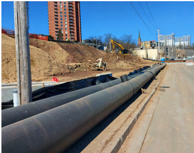
Cogswell District Energy System Lines Prepared for Installation
