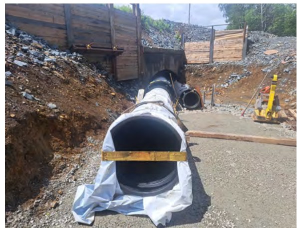
Churchill Drive Water Transmission Main Replacement
