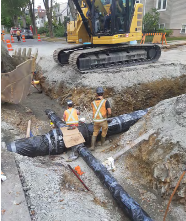
Dublin Street Water Transmission Main Upgrade
