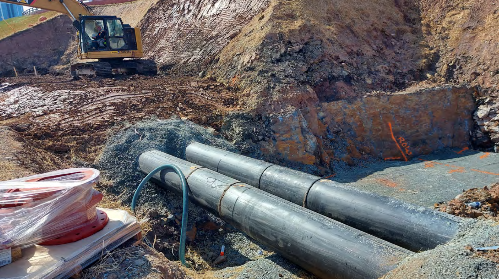
Cogswell District Energy System Lines Being Installed
