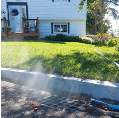
Manhole smoke test
