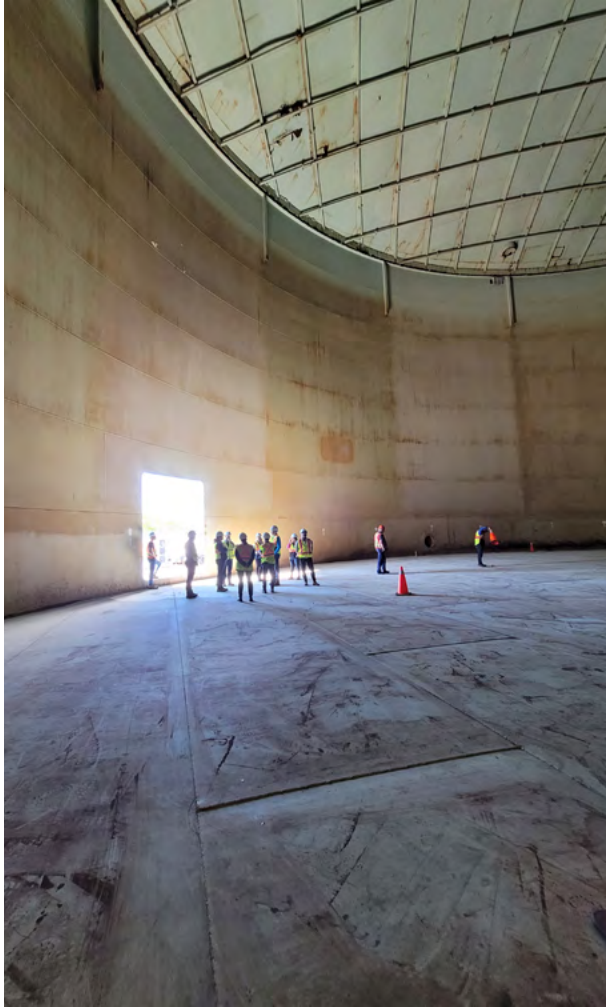
Inside the Akerley Reservoir
