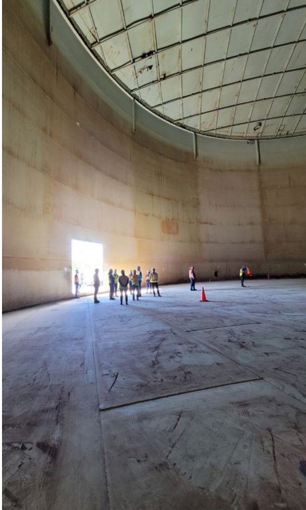
Inside the Akerley Reservoir
