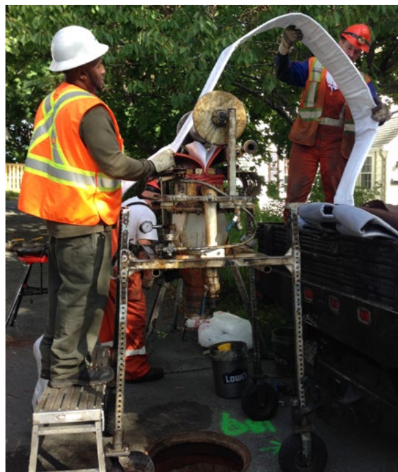
Cured-In-Place Pipe Lining Work Reducing Wet Weather Flows
