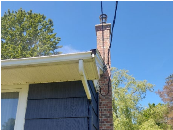
Private downspout smoke test
