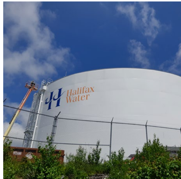
Akerley Reservoir - After
