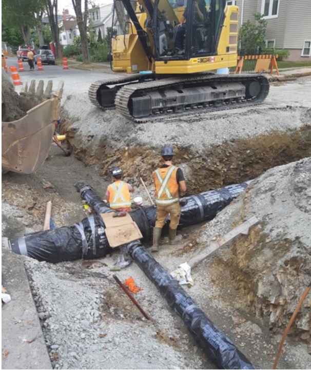
Dublin Street Water Transmission Main Upgrade
