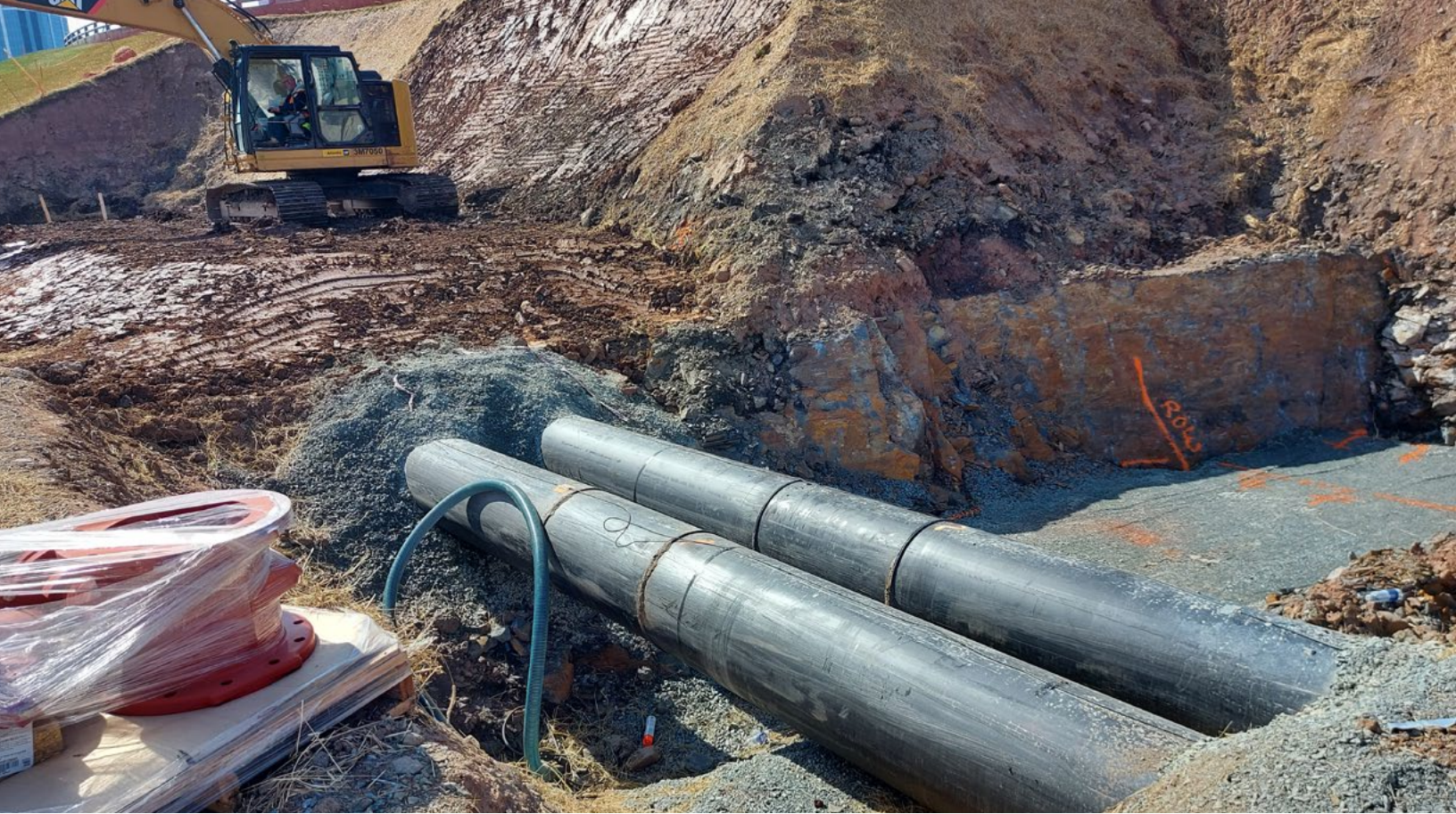
Cogswell District Energy System Lines Being Installed
