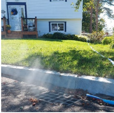
Manhole smoke test
