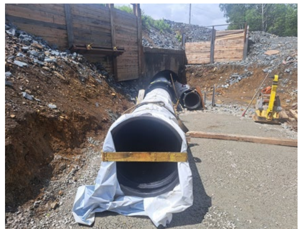
Churchill Drive Water Transmission Main Replacement
