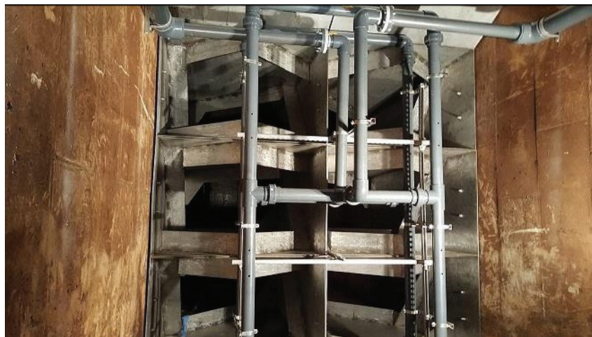
Figure 3.1: In-Channel Static Mixer
