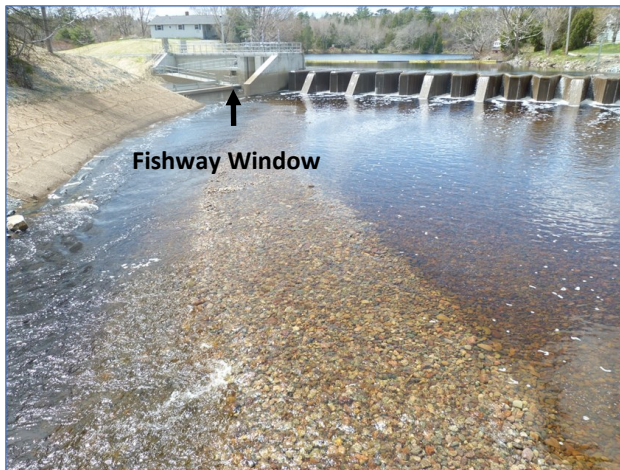
New Lake Major Dam and Fishway
