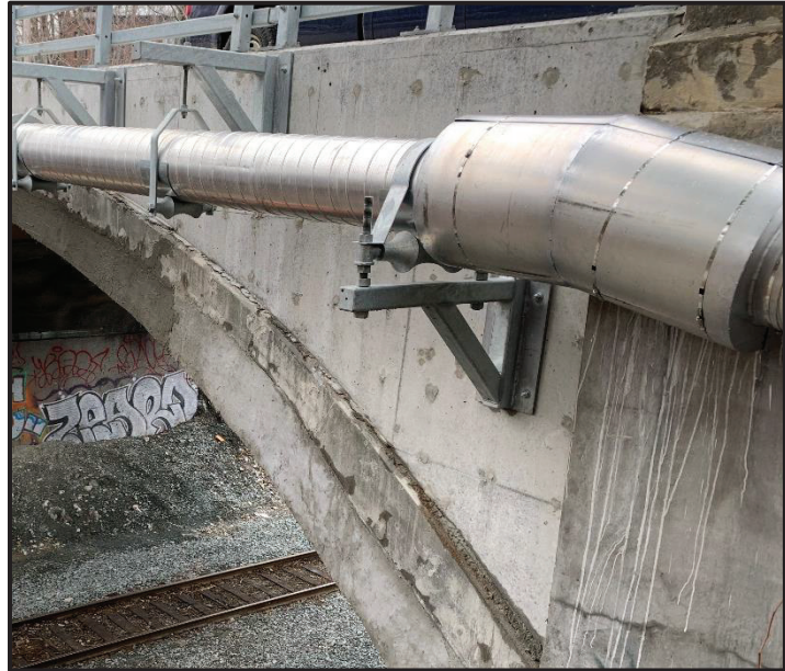
Figure 4-6: Watermain Support Hangers at Marlborough in 2019
