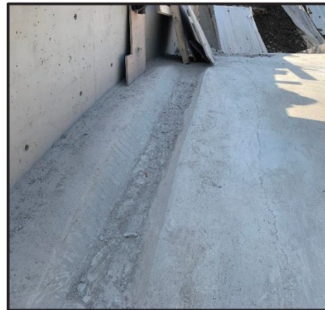
Figure 4-3: Depression in Arch at Coburg Bridge in 2020
