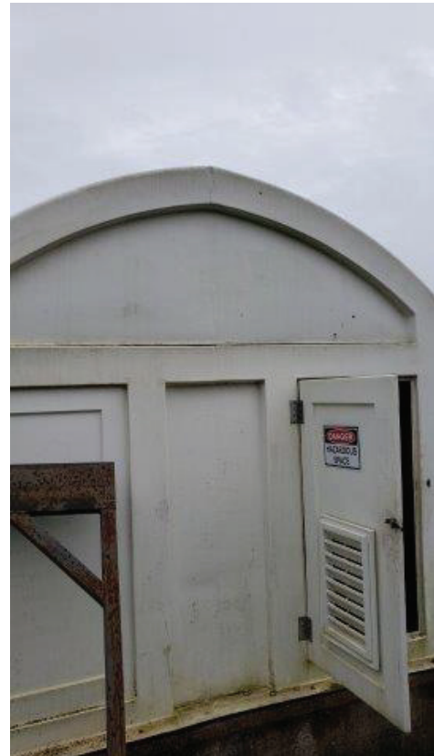
B10: Access door to rear of building. Slight damage to FRP covers.
