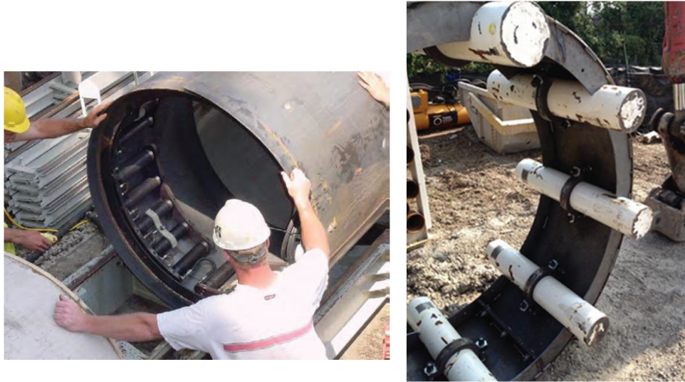
Figure 2 Intermediate Jacking Station
