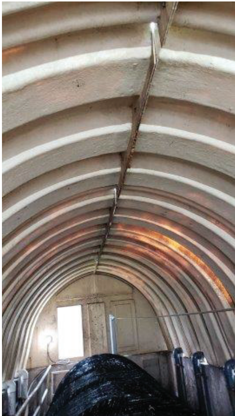
B13: Joint ridge in FRP covers – not weather tight
