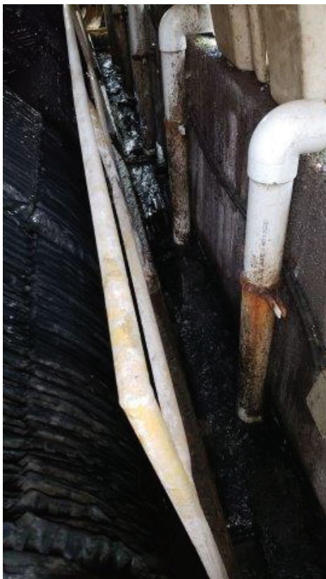
B15: Desludging pipe inside RBC and notable build-up of surface scum.
