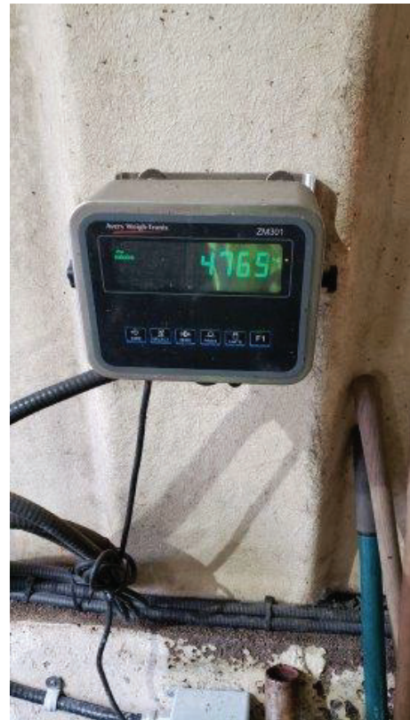
B6: Load cell display – not hazardous rated.
