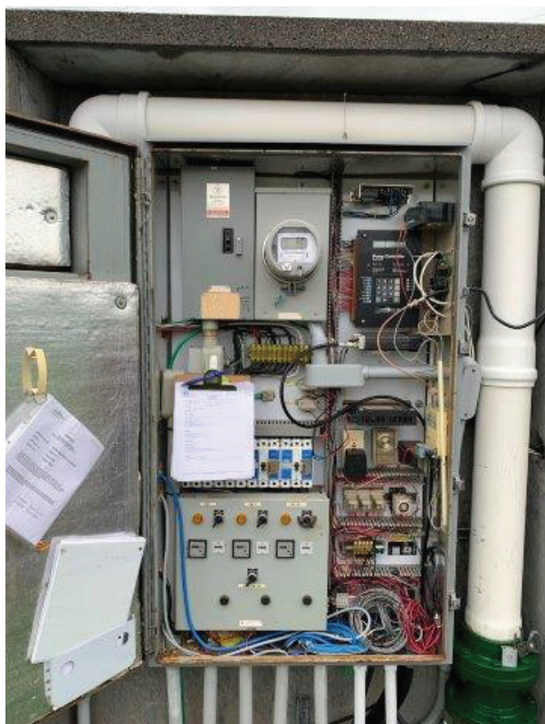
B1: Main distribution panel. Conduits not sealed, and components corroded, aged, and outdated.
