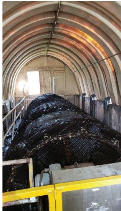
B14: RBC media – damaged and steel supports corroded.
