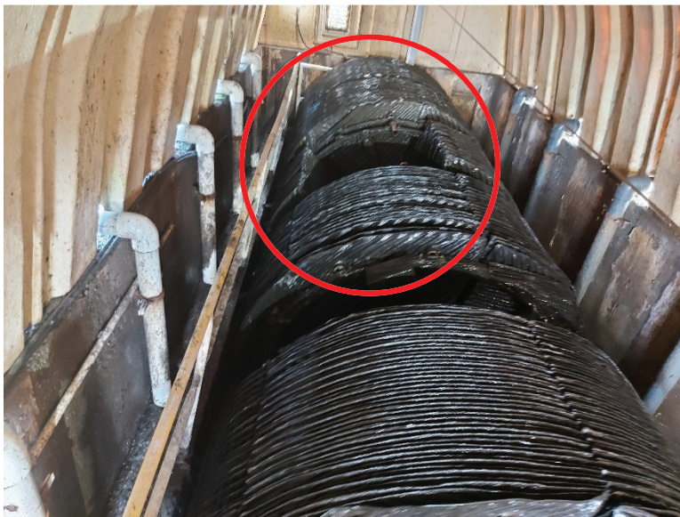
Figure 2 - Deteriorated and Missing RBC Media and Supports.
