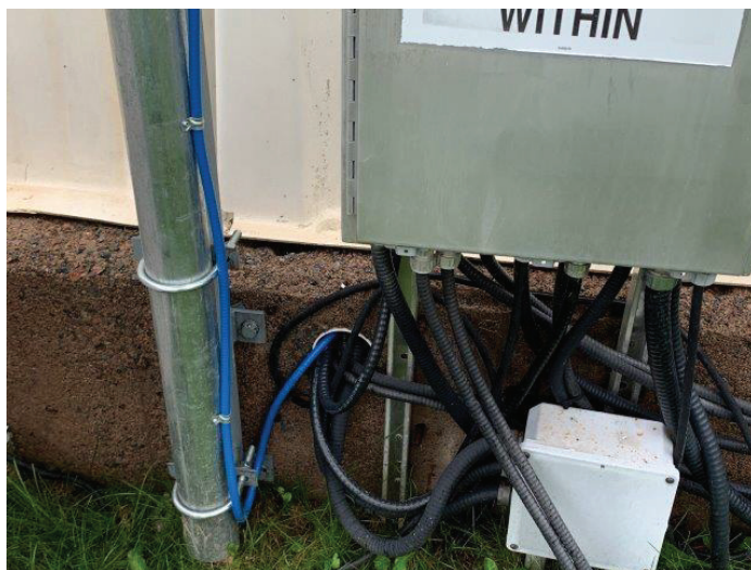
B2: Cable conduits not sealed.
