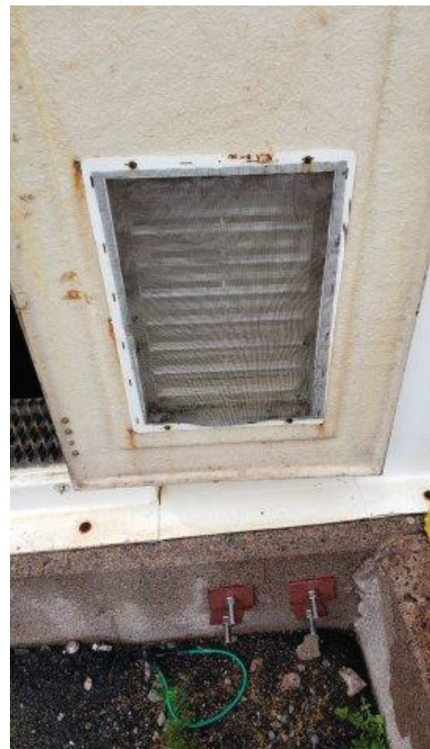
B12: Existing air intake louver – showing signs of corrosion.
