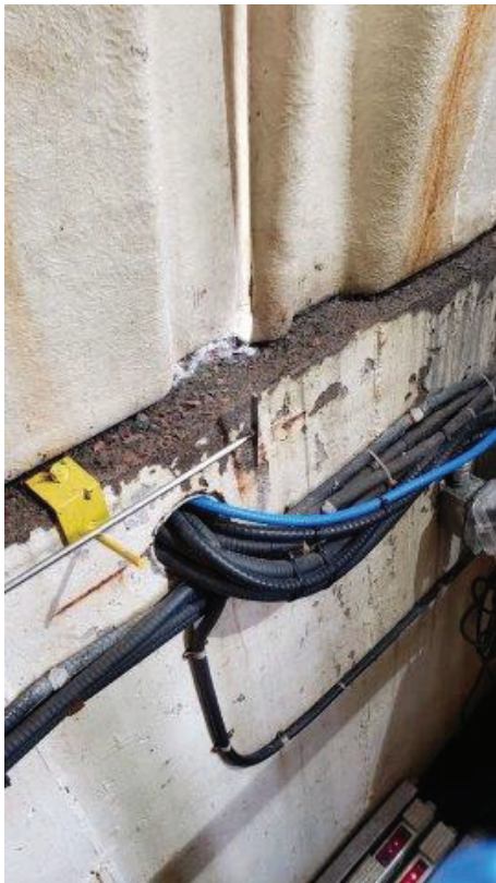
B5: Cable wall penetrations not sealed.
