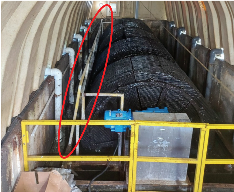
Figure 1 - Safety Rail on One Side and in Poor Condition.
