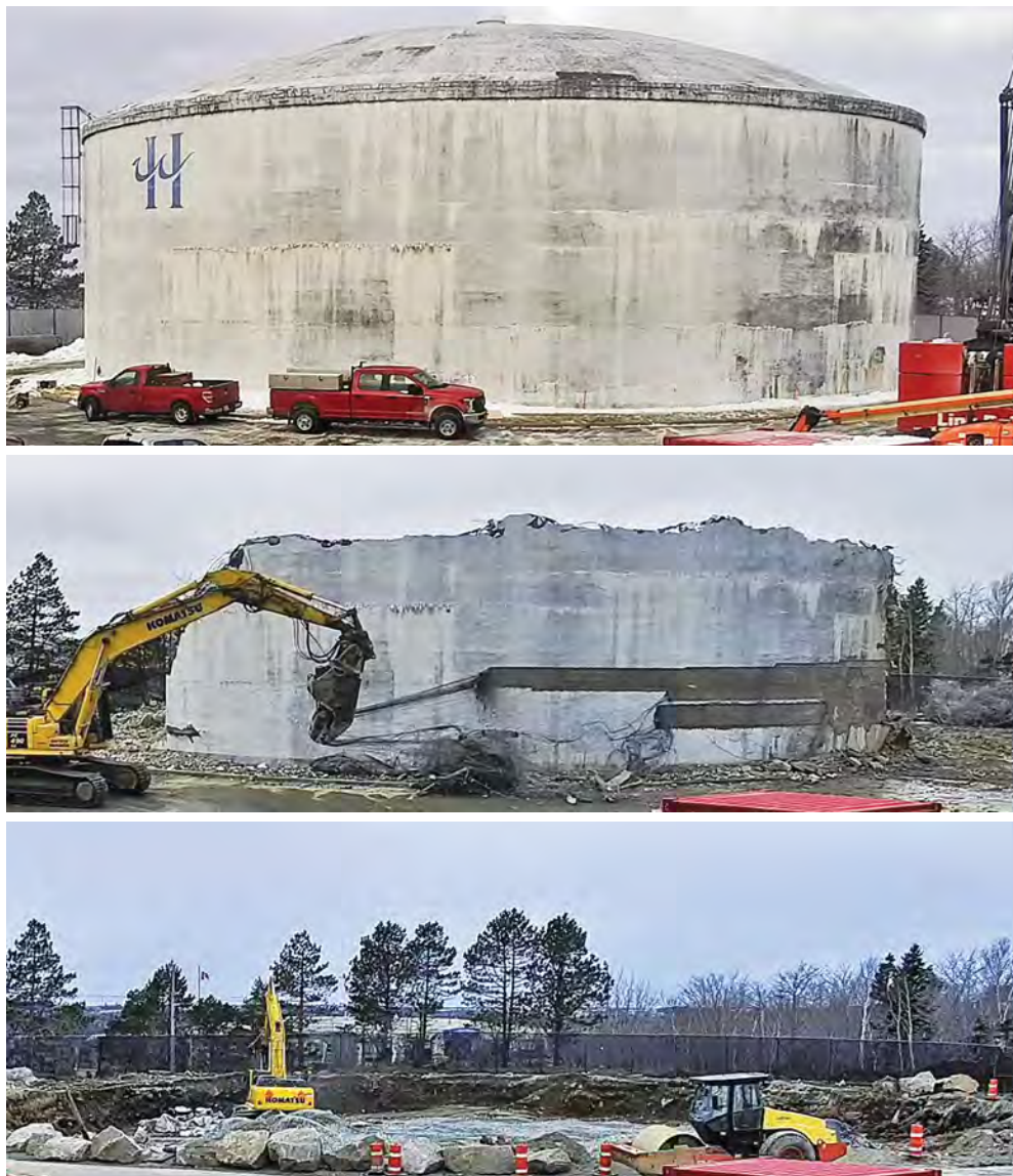
The demolition of the old Cowie Reservoir in preparation for the construction of a new reservoir in its place.
