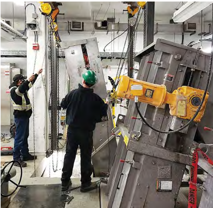
Figure 7: Installing Fine Screen No. 3 at DWWTF.
