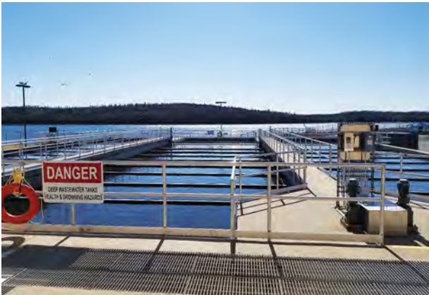
Secondary clarifiers automatically come online and offline according to defined flow ranges.
