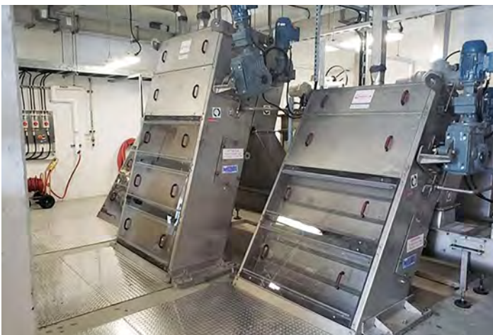
Figure 8: Completed screens installed at DWWTF.
