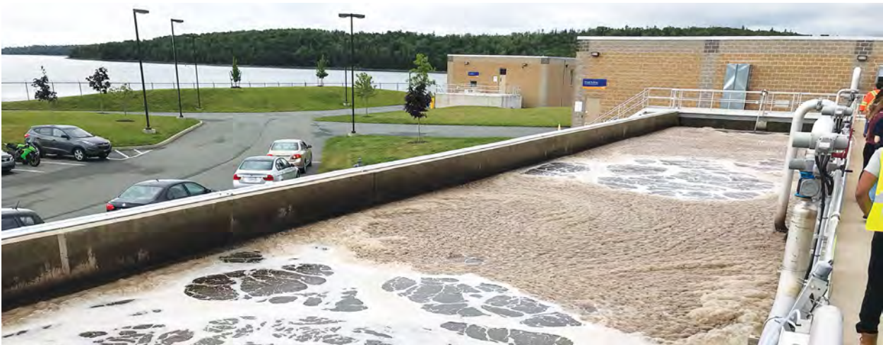
Three aeration tanks where microorganisms are conditioned to good health before fully coming online to treat high wet weather flows.
