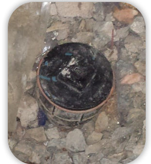
Typical Cleanout Configurations (Generally a 10 cm (4") diameter pipe in the basement.)
