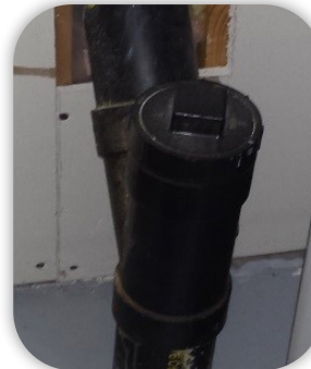
Typical Cleanout Configurations (Generally a 10 cm (4") diameter pipe in the basement.)
