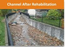
restoration efforts of this project will use energy dissipation pools, natural pool and riffle sequencing and natural stone on the bottom of the channel liner. This provides a naturalized stream bottom that reduces velocities, creates pools and meanders and helps to improve fish passage.
