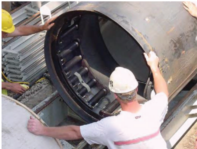
Figure 7 Intermediate Jacking Station
