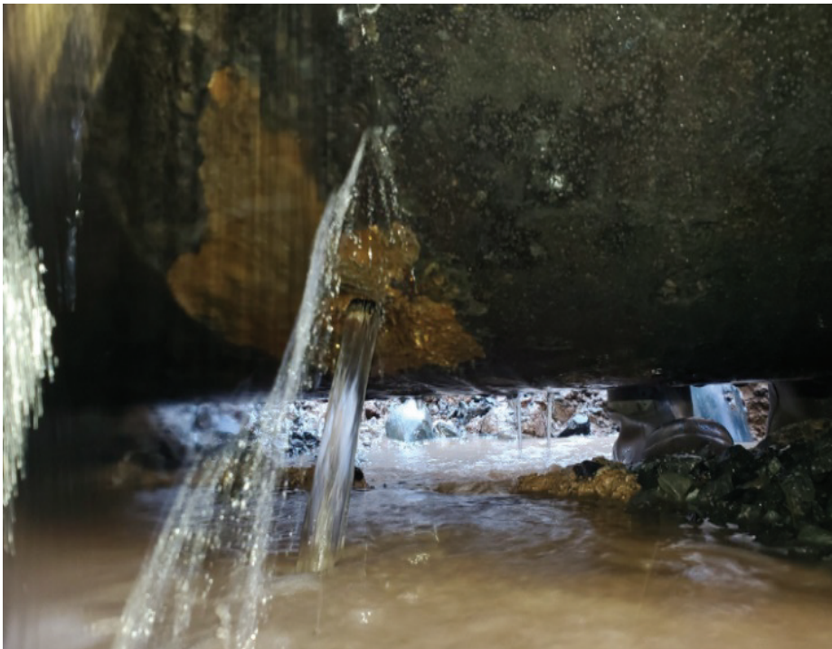
Fig. 4a – Hole in Pipe
