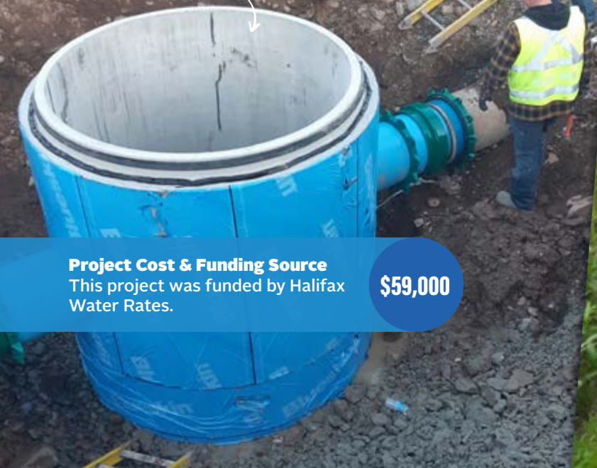
New 1800 mm Chamber Installed
