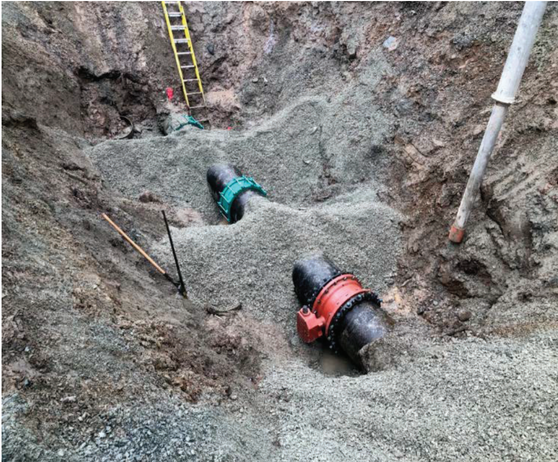
Fig. 4c – New Pipe and Valve
