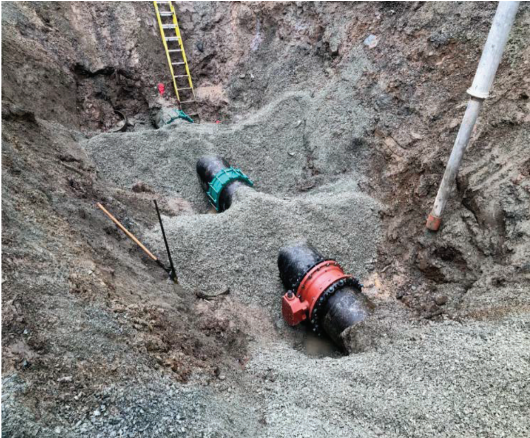
Fig. 4c – New Pipe and Valve
