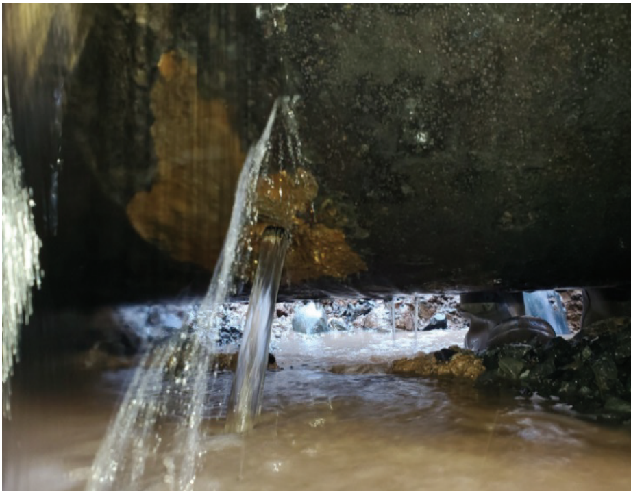
Fig. 4a – Hole in Pipe
