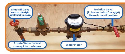
To do this, **turn your shut-off valve into the "Closed" or "Off" position.** Either the shut-off valve or the isolation valve, once closed, will prevent water from leaving your home. (If either valve is seized or malfunctioning, a plumber should be contacted to repair or replace the valve. These valves are the responsibility of the property owner.)
