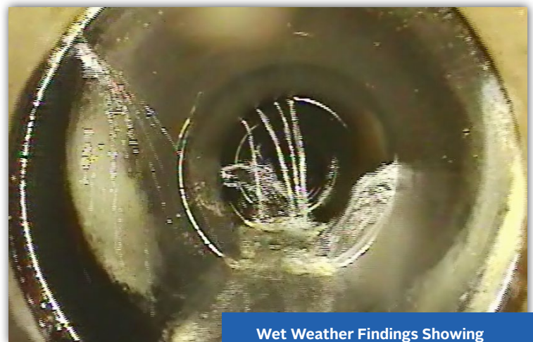
Wet Weather Findings Showing Stormwater Infiltration at Pipe Joints
