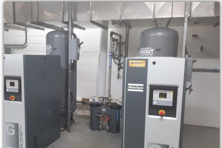
New, efficient air compressors installed at the Halifax WWTF
