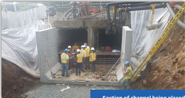
Section of channel being placed
