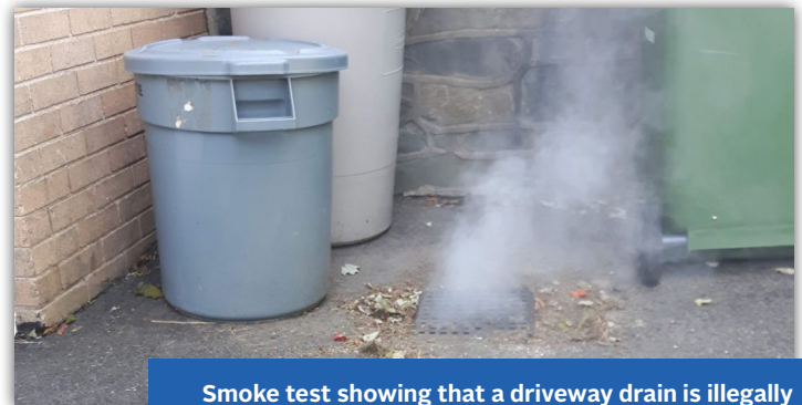
Smoke test showing that a driveway drain is illegally connected to the Halifax Water wastewater system
