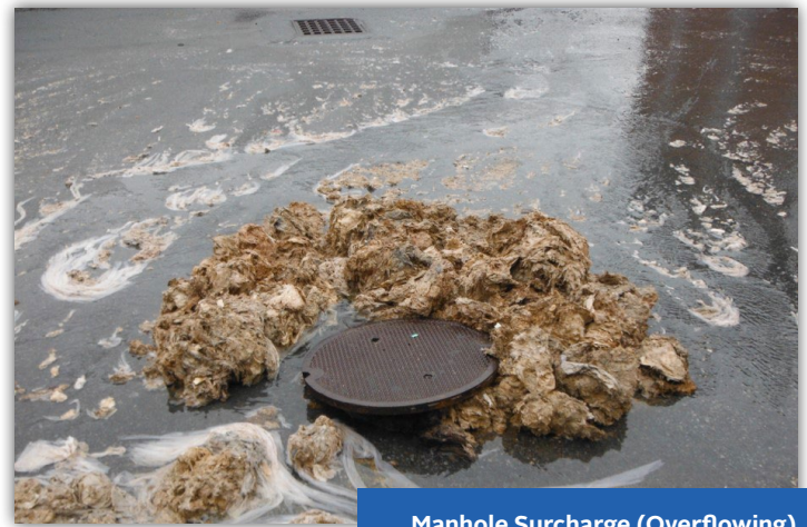
Manhole Surcharge (Overflowing)
