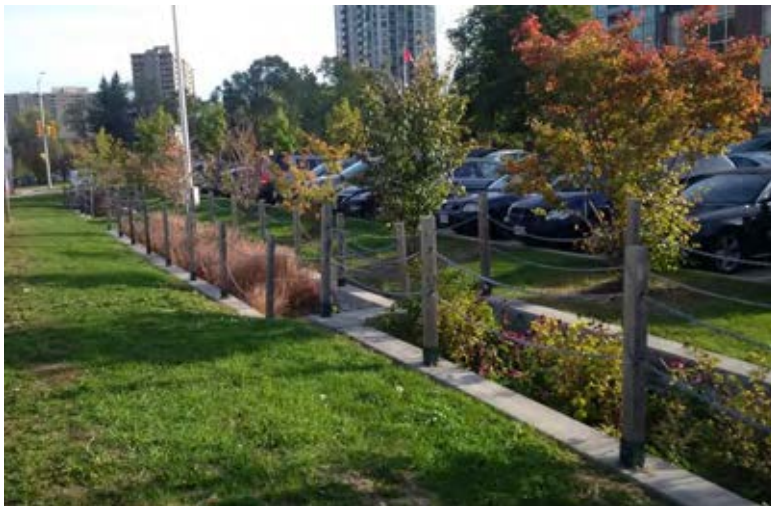
Figure 3: Rain Garden Boxes for Storage, Infiltration, and Water Quality
