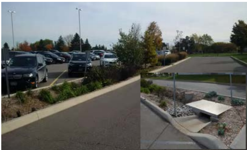
Figure 6: Private Parking Lot – Permeable Pavers and Bioswale
