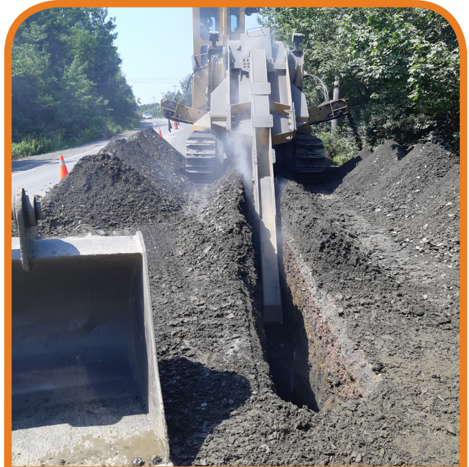
Trenching machine cutting down through asphalt, rock, gravel and dirt to begin the excavation work for the new water transmission main.
