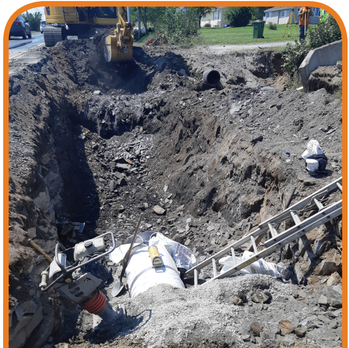
New section of water transmission main installed and partially backfilled, excavation continues to prepare for the installation of the next section.
