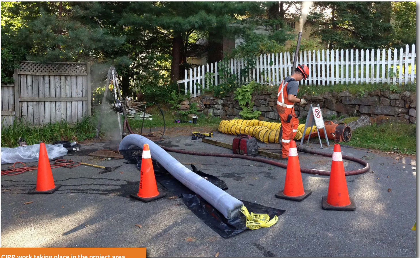
CIPP work taking place in the project area
