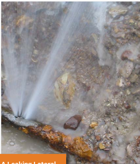
A Leaking Lateral
