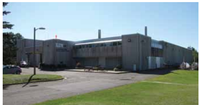
Pockwock (J.D. Kline) Water Supply Plant
