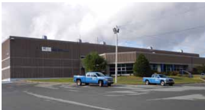
Lake Major Water Supply Plant
