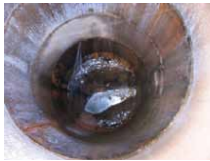
Leaking pipes lead to added costs and possible sewage overflows
