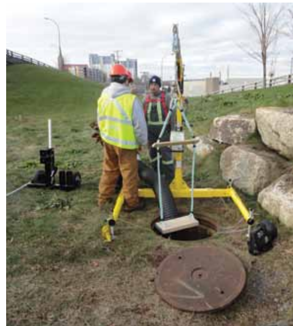
Proper training and equipment for a confined space entry
