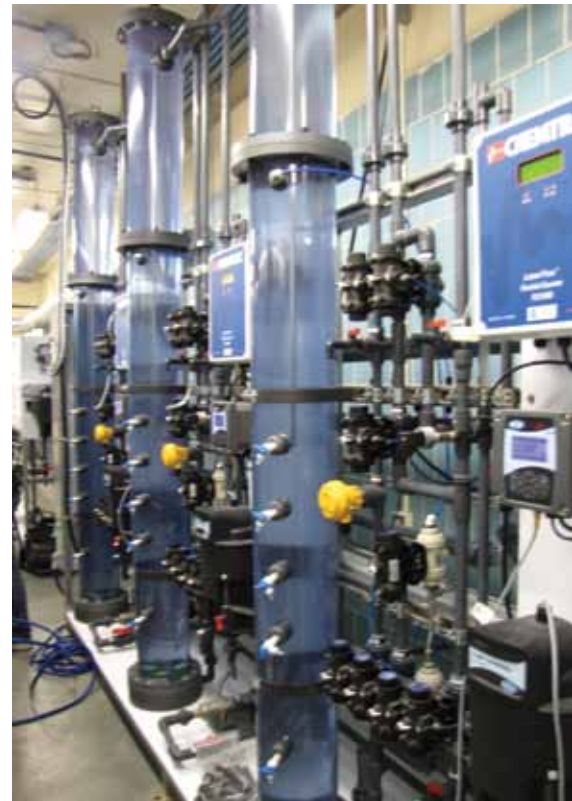
Pockwock Pilot Plant – water research in action
