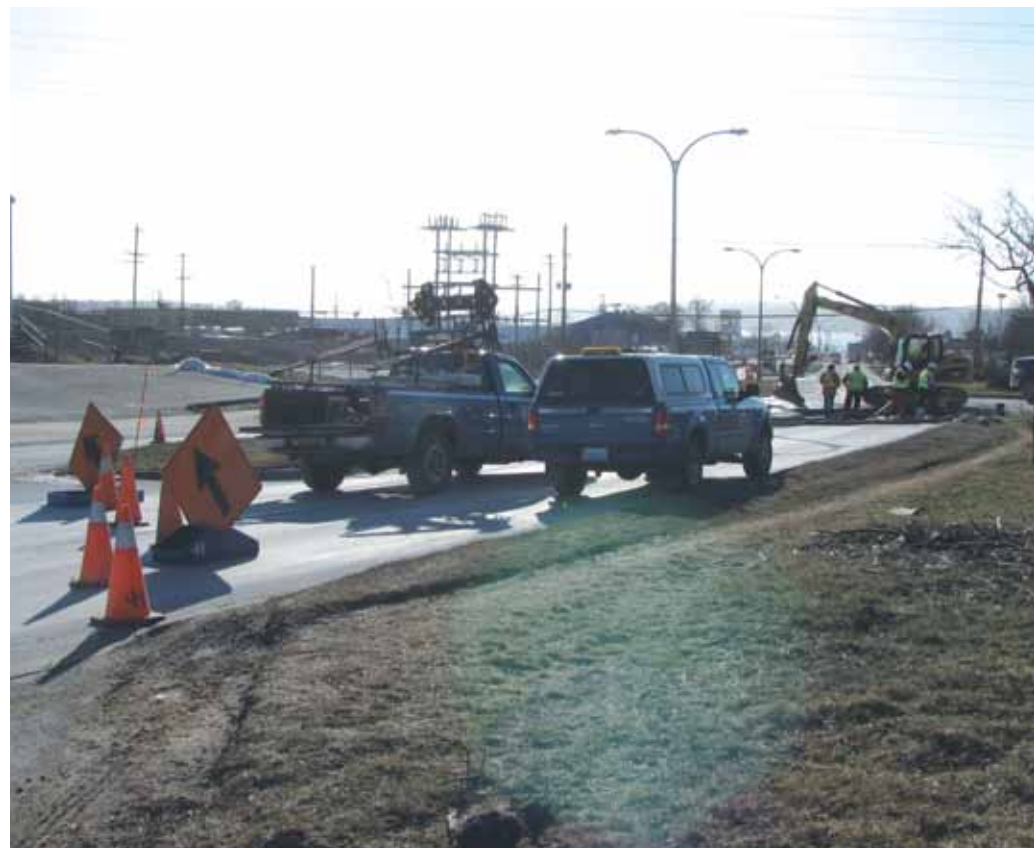
Proper traffic control for the safety of the public and Halifax Water staff
