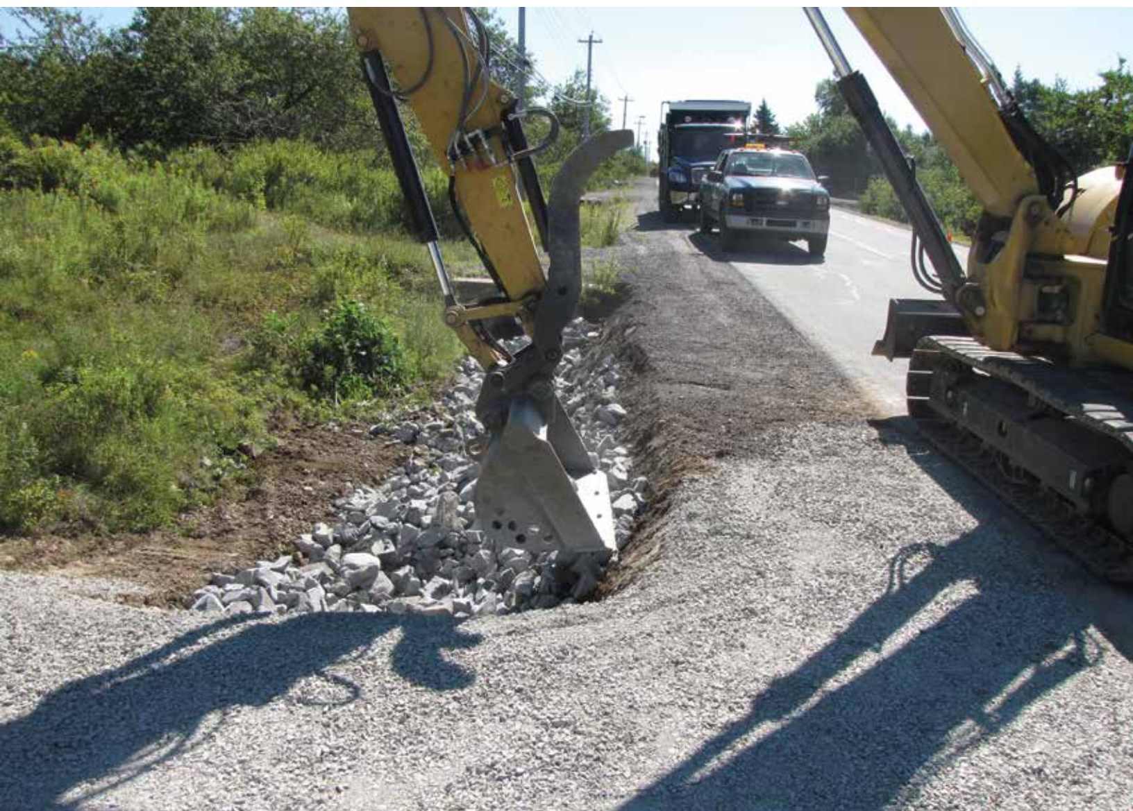
Ditch and culvert repair to improve stormwater service for the community of Hammonds Plains
