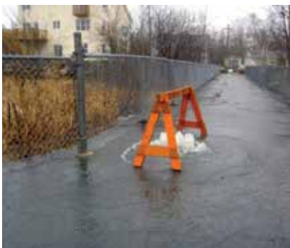
The result of excess stormwater in the wastewater system – a system surcharging
