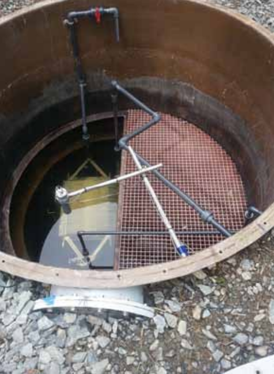
Frame WWTF producing high quality effluent
