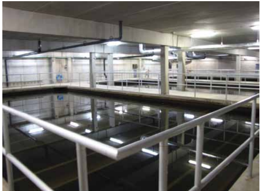
Pockwock water treatment facility, filter gallery
