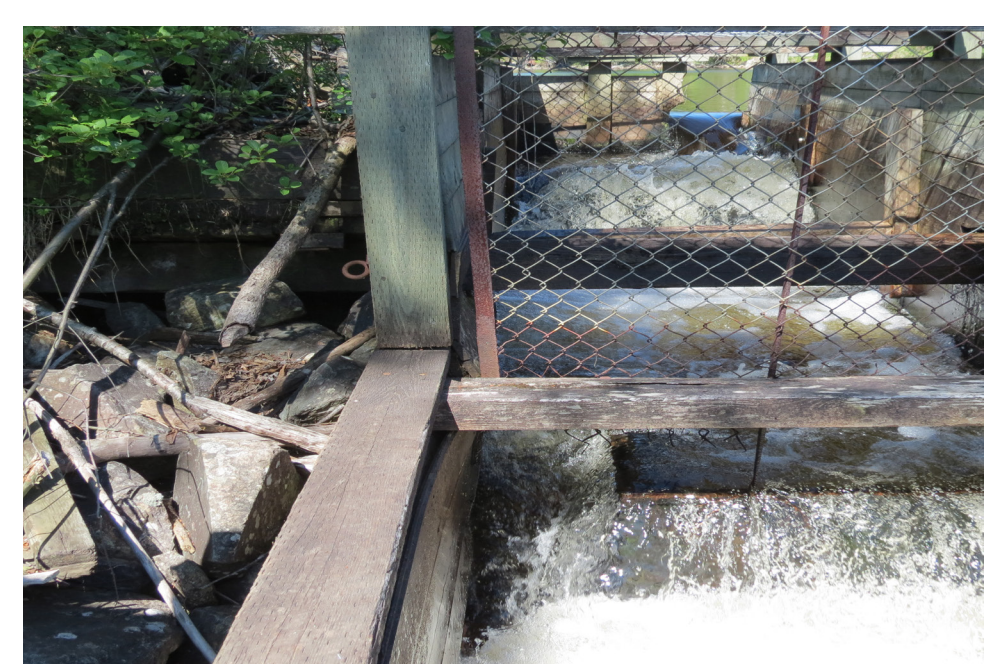
ORIGINAL FISHWAY IN OPERATION
