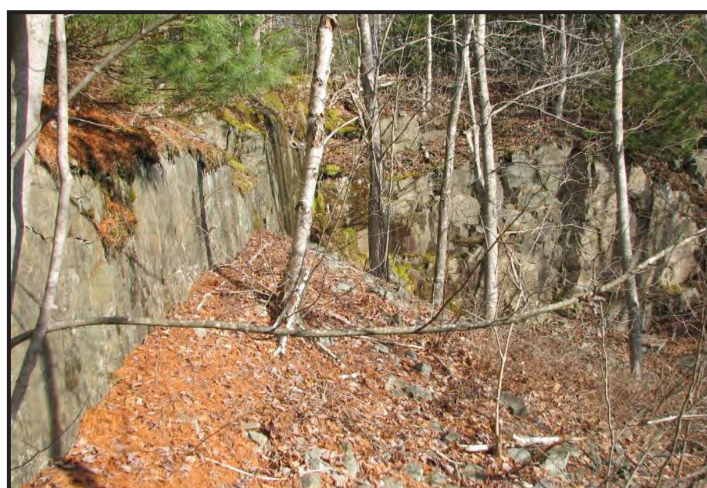
EVIDENCE OF HISTORICAL QUARRY
