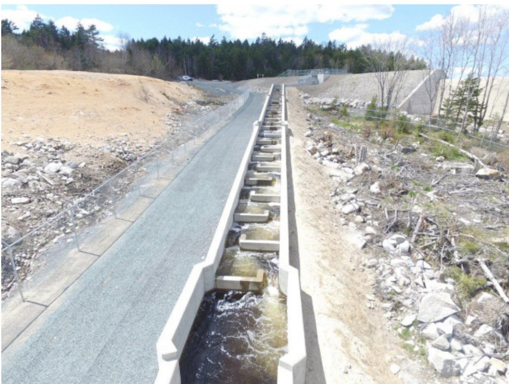
EXAMPLE POOL AND WEIR FISH LADDER AT SANDY LAKE DAM
