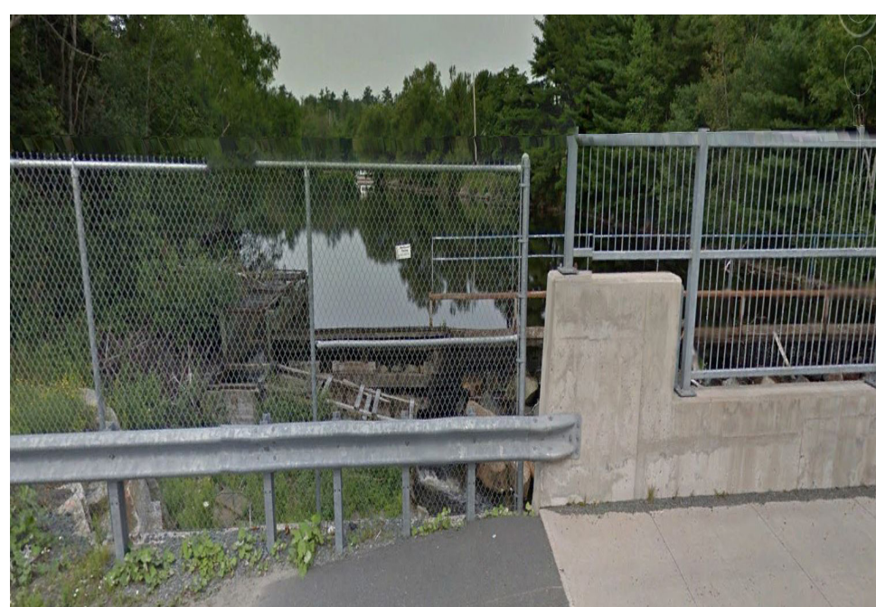
IMAGE OF DAM FROM BRIDGE Credit: Google Earth
