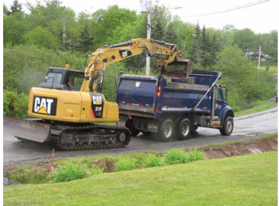
Performing ditch maintenance to effectively manage stormwater drainage
