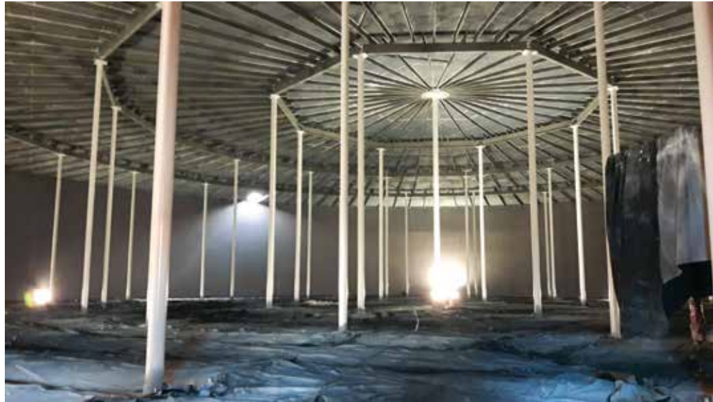
Painting the interior walls and columns at the Geizer 158 Reservoir
