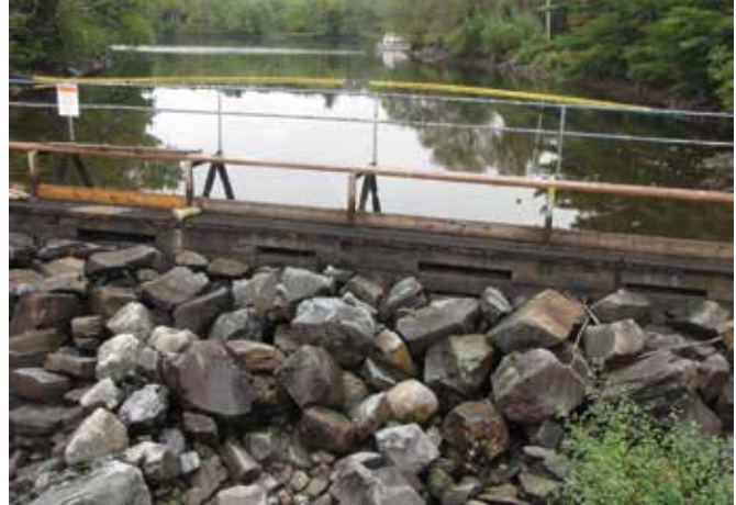
Lake Major Dam September 14, 2016
