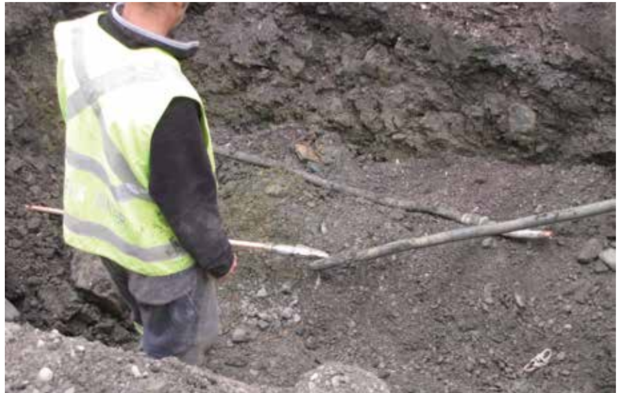
Halifax Water replacing a lead service line with a new copper line
