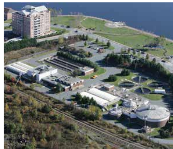
The Mill Cove WWTF—part of the community since 1969
