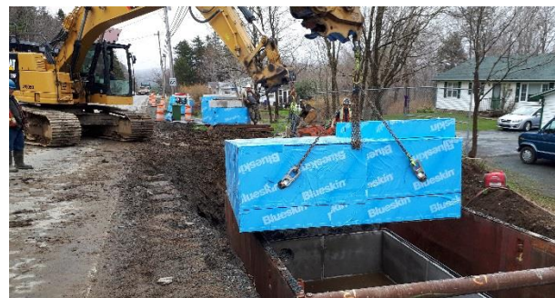
A Pressure Reducing Valve Chamber being installed on Fall River Road.
