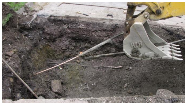
Backhoe removing a lead service line.
