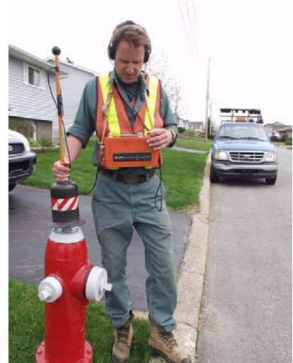
Acoustic Leak Detection Equipment being used to pinpoint a leak between hydrants.
