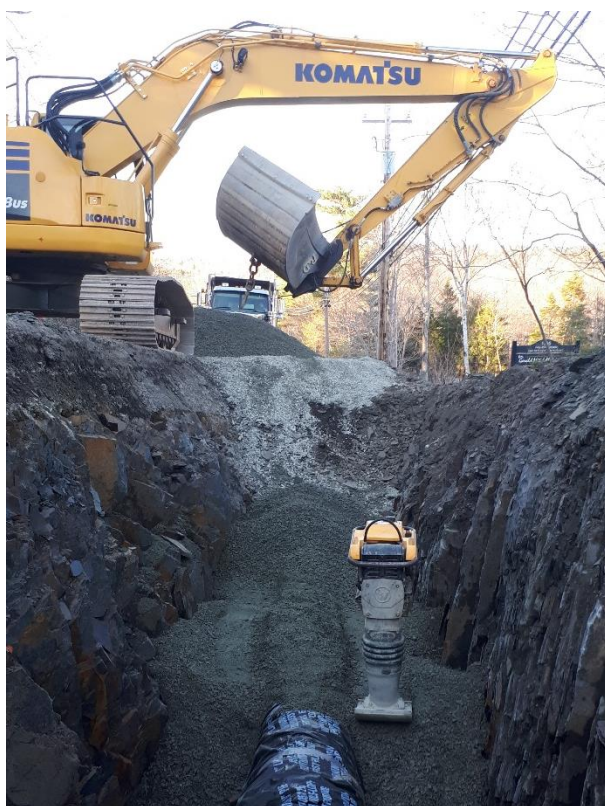
A section of water main being installed on Fall River Road.
