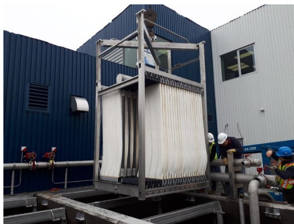
Installation of the membrane modules.
