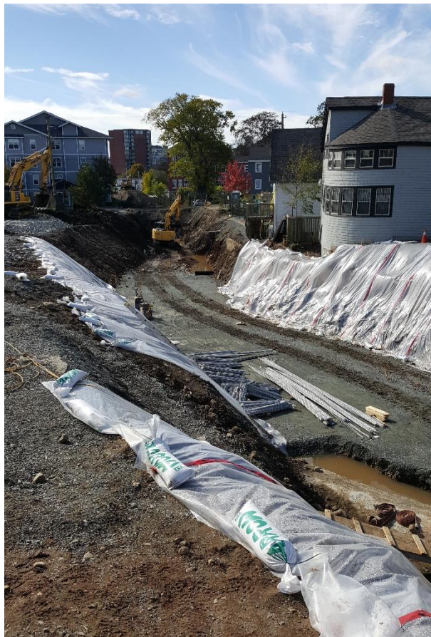
Sullivan's Pond – Construction of new open-channel.
