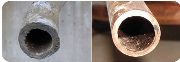
Left: Lead Service Line, Right: Copper Service Line.
