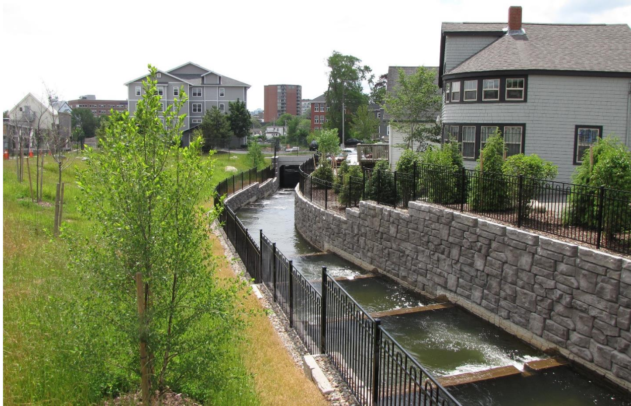
Sullivan's Pond – Completed section of open-channel. Final landscaping work underway.
