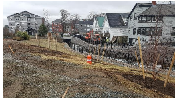
Sullivan's Pond – Construction of new open-channel.
