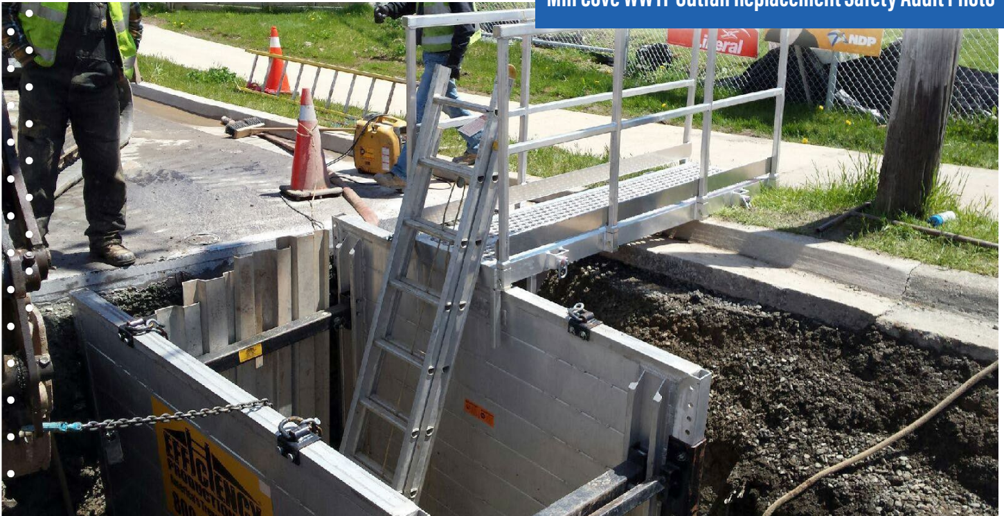
Fall River Water Service Extension Safety Audit
